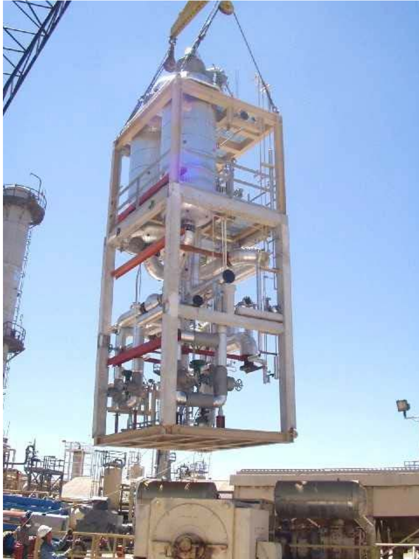
Figure 4 The IsoTherming Unit Ready to be Set
